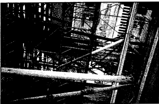
Horizontal supports to the scaffolding were examined and evaluated.
