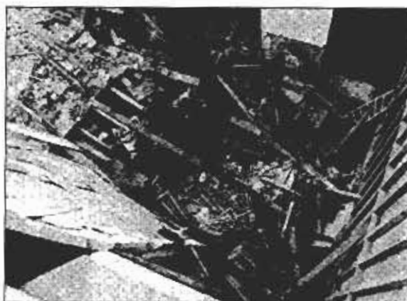
Three floors of the structure tumbled, pancake fashion, and came to rest on the first floor. All hope of rescuing the victim (center) rested on the possibility that individual voids had been formed by the unstable debris.
